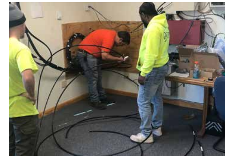
Workers splice new fiber optic cable on Washington Island.
