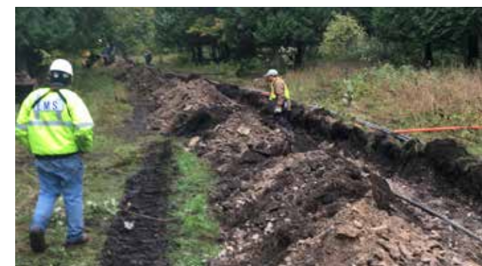
A crew installs the new underground power cable across Plum Island.
