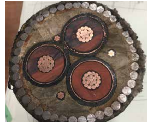
A section of the old submarine power cable.
