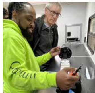
Clinton Triplett, of contractor Quantum Technology, provides a fiber optic fusion splicing demonstration for Governor Evers during the governor's visit to the Washington Island Electric Cooperative.
