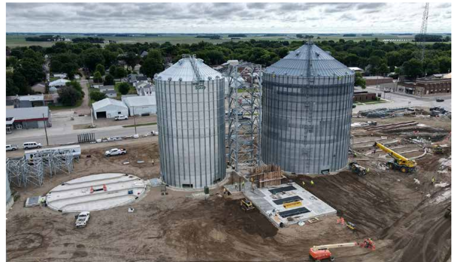
Grain bins in place after being moved to new foundations.
