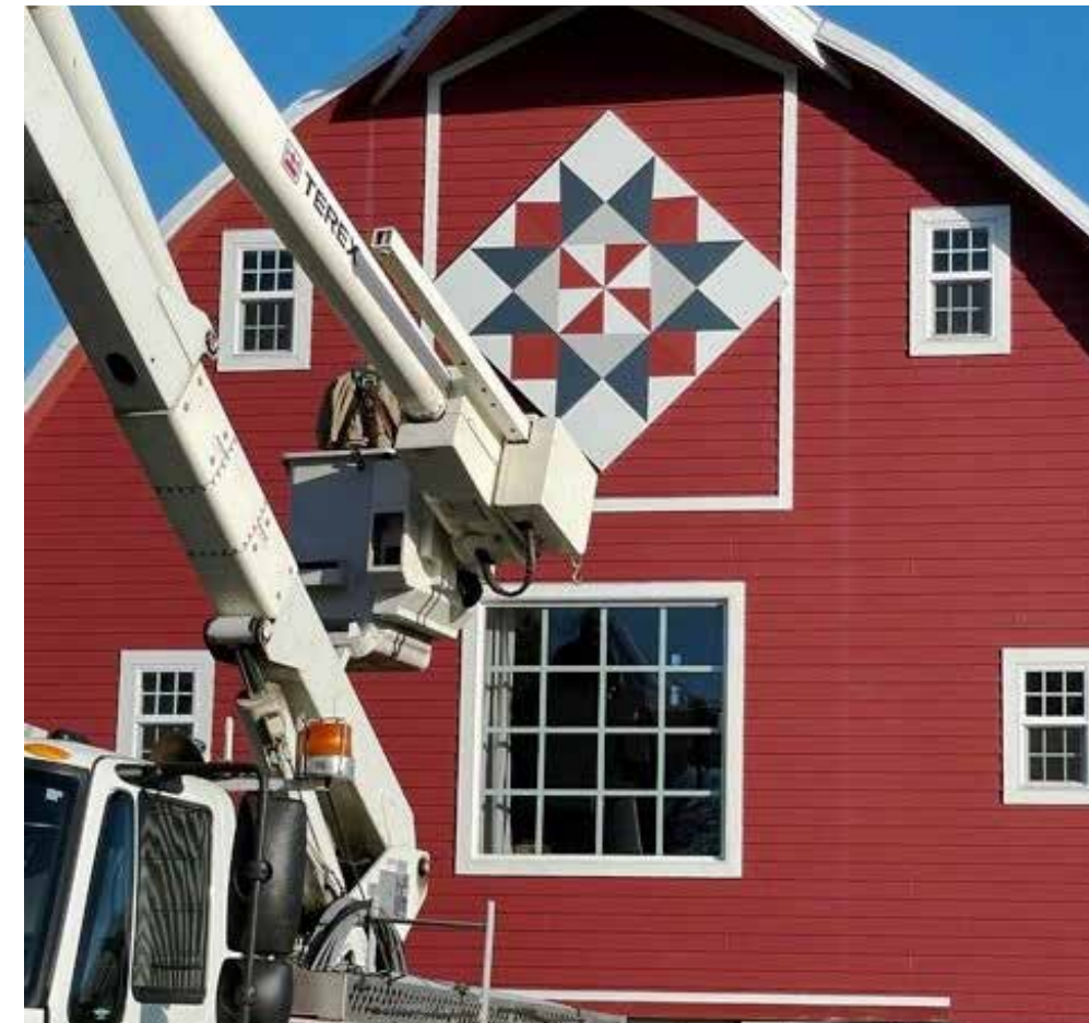
A Todd-Wadena bucket truck was key to hanging this quilt on the side of a barn. (Photo: Todd-Wadena Electric Cooperative)
